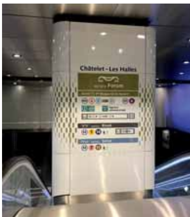
Habillage architectural en émail, RATP Station Châtelet les Halles, Paris [75]
